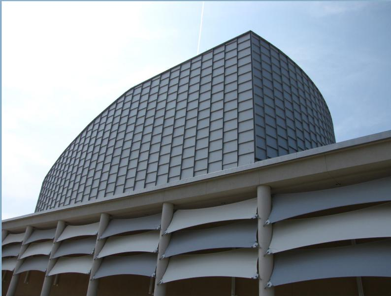
InvariMatte® stands by itself as the premium roofing material. Its high reflectivity of solar radiation gives it the industry's highest SRI of 113, when measured using the alternative method to that used for painted surfaces. Its unique self-cleaning surface and resistance to corrosion keep that SRI at the same level for over 10 years without cleaning or maintenance. Despite this, it is not shiny; it has a gloss near less than that of some paint finishes. How does it do this?
