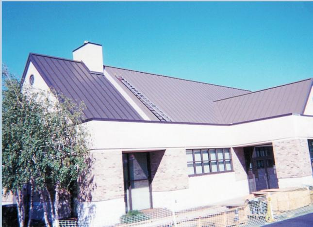
Since stainless steel has a melting point about 2800°F, it is very unlikely that airborne cinders coming in contact with the stainless steel roof, for example will ignite a fire. Except for carbon steel which has a similar melting point, the other metals used in construction have melting points that range from 500 to 1200°F.
